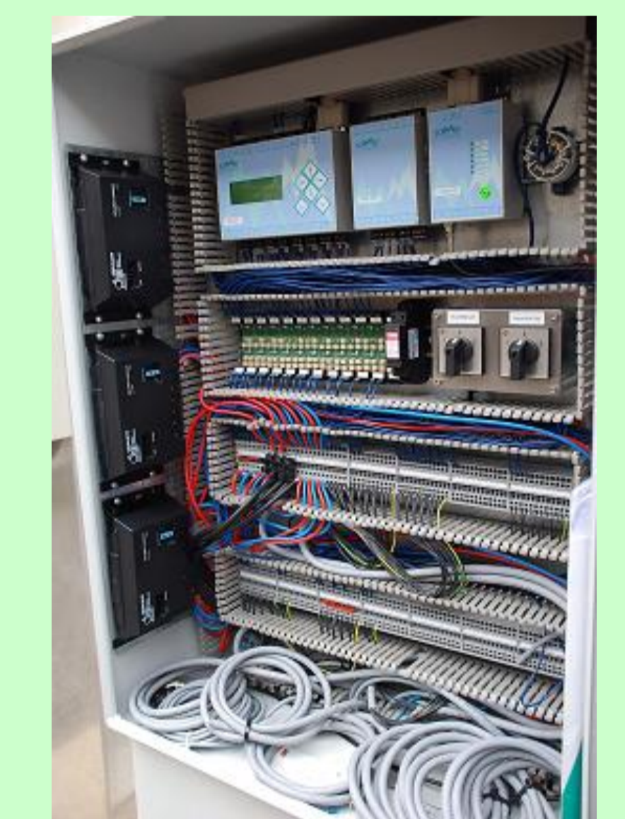
Figure 6: Electronic control box with data logger and radio transmission unit, will be lifted.
