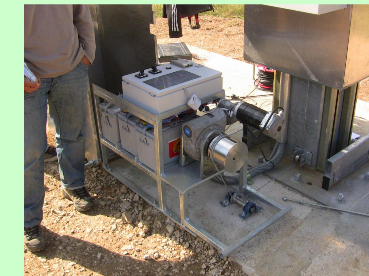
Figure 5: Accu, lifting control box, electromotor and winch. All components are fixed at the ground.
